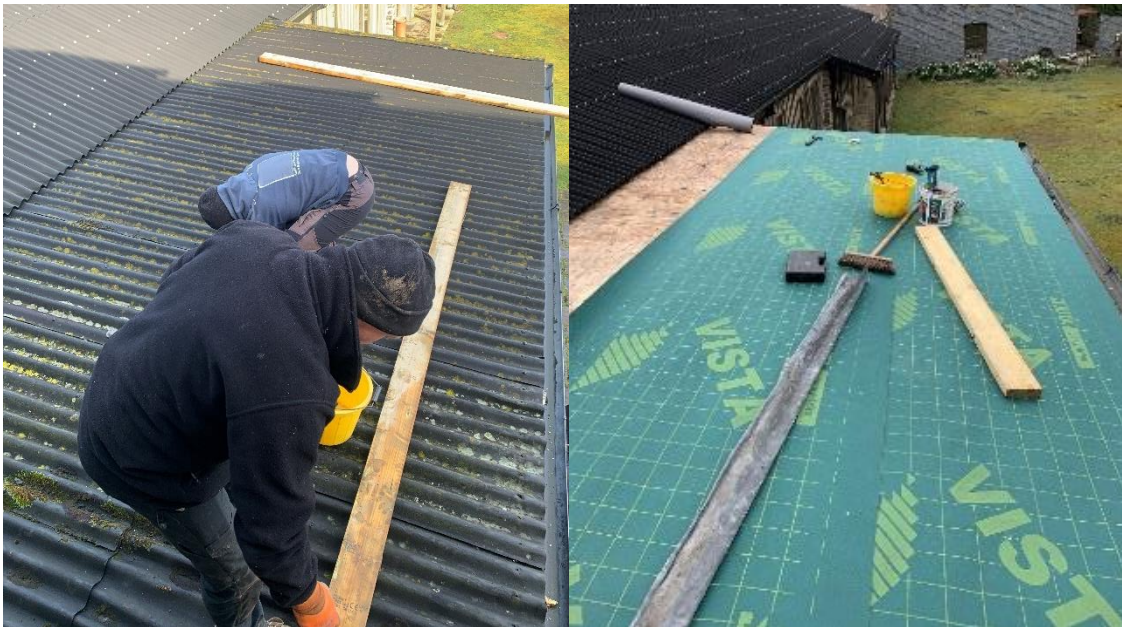
Battery room roof replacement in progress
