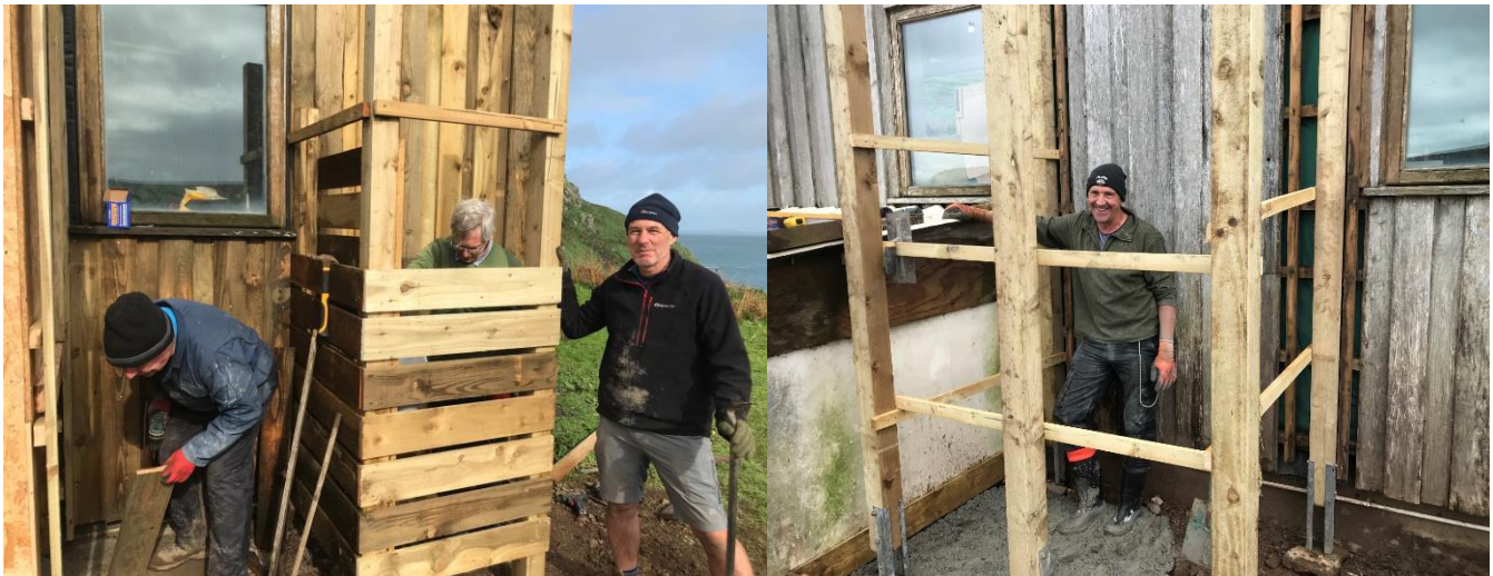
Autumn Work Party building compost toilet and urinal.
